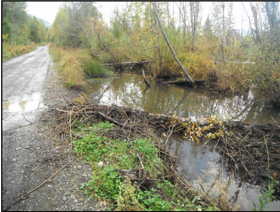
Photo 4: Looking west on 26-Mile FSR, typical beaver dam requiring breaching to prevent water from flooding the road (taken September 24, 2012).
