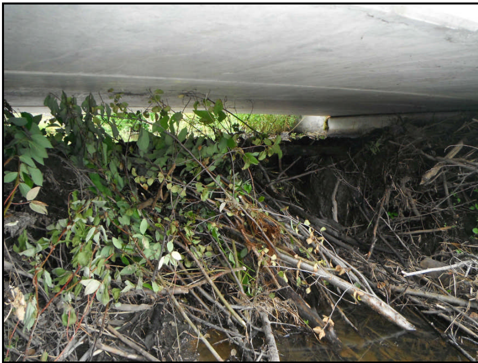
Photo 1: August 14th, 2012. Looking upstream under the bridge at km 3 on the 26-Mile FSR, before breaching.
